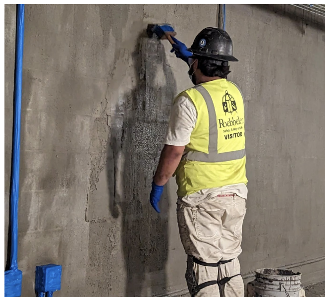
Megamix 1 and Xycrylic Admix being sprayed on the wall.
